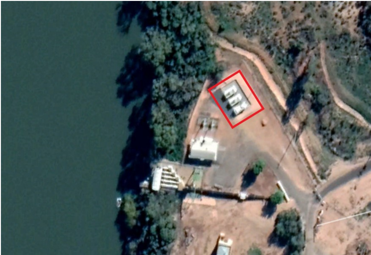
Figure 2: Location of Generators and Diesel Fuel Tank
