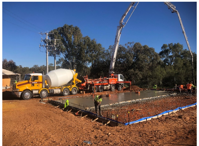
Concrete slab being poured at the Coomealla pump station for the 2 generators and fuel tank.
