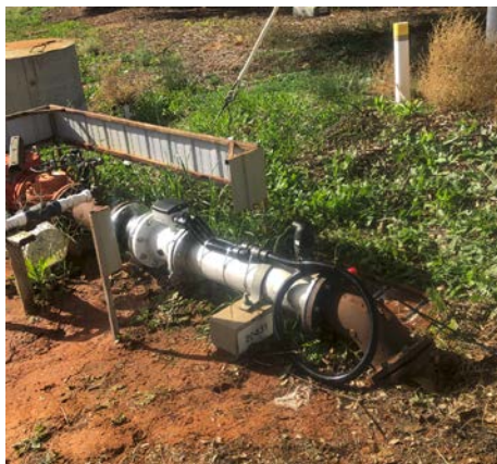
Replaced meter awaiting telemetry pole Telemetry pole
